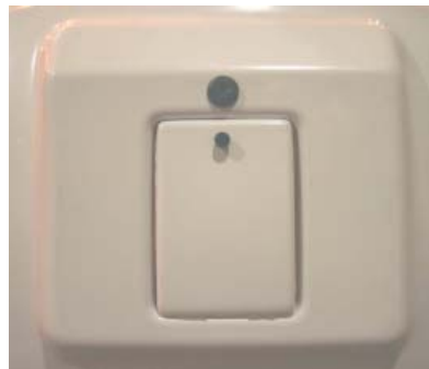
Figure 26 - Fuse Access Panel
